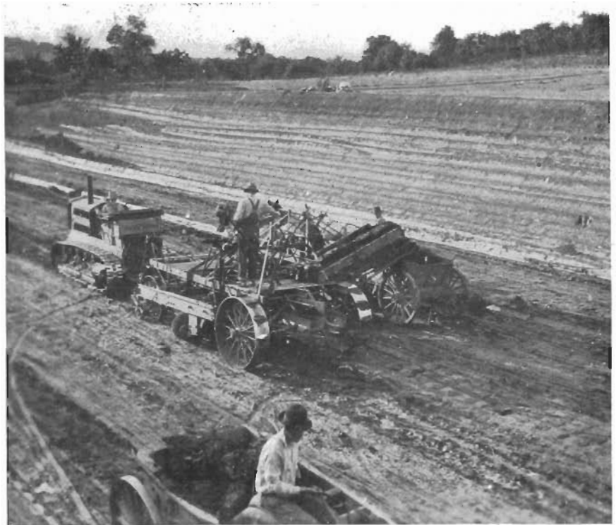
This photograph might be carded, the only sure way to fix railroad crossings—tunnel under.
