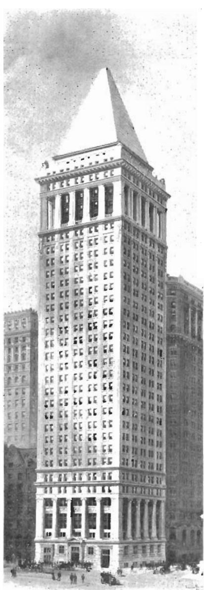
development of the principle applied in cofferdam foundation work under the Mutual Life & Commercial Building
