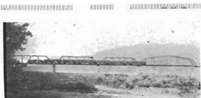
Train 715 crossing the Frisco Fort Smith-Van Buren Bridge.
