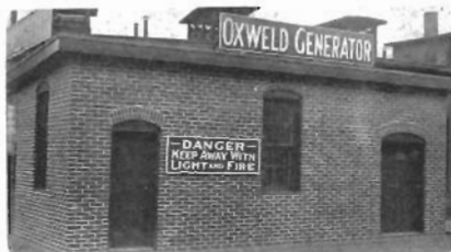
Oxy Acetylene Generator Plant, Kansas City, Mo.
