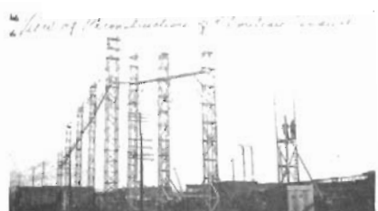
View of Choteau Viaduct Reconstruction
