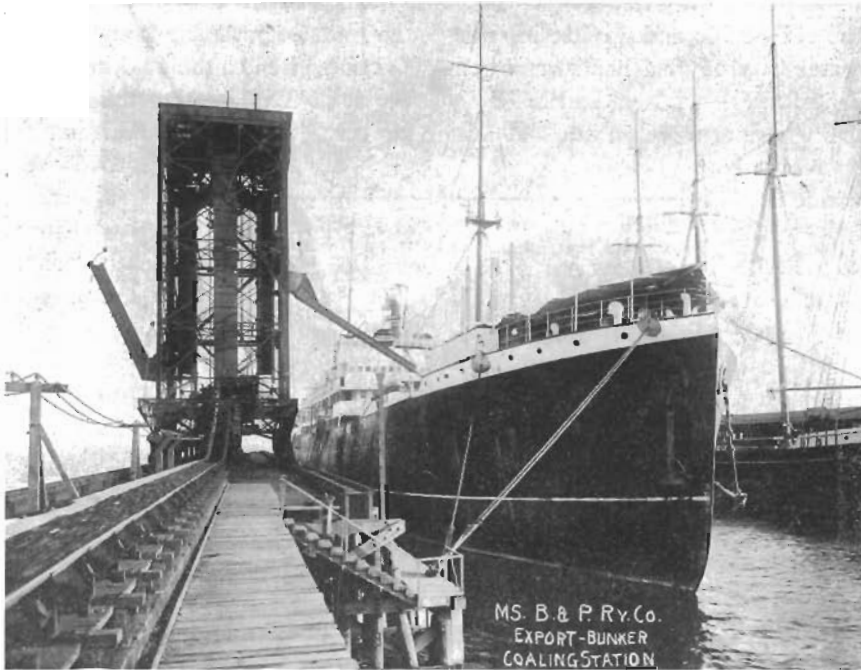
The immense coal tippie of the M. S. B. & P. Railroad Company at Pensacola, Florida, in operation
