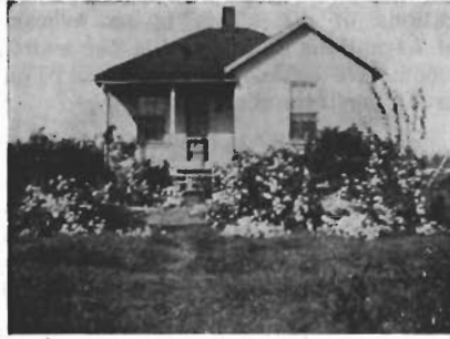
A picture of the section house and yard at Frenchman's Bayou, Ark., taken by James W. Williams, section foreman at that point. "This is what we had in the way of flowers around our section house in 1927, and we hope to make it still more beautiful in 1928," writes Mr. Williams.
