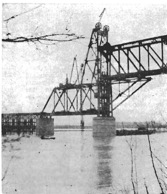
The Warrior River bridge lift span under construction showing the temporary bracket support.
